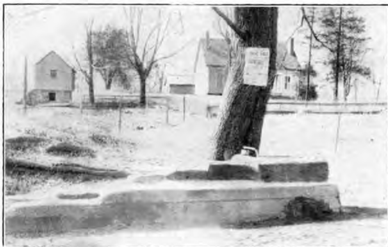
One of Vermillion County's big springs improved for public service. A favorite spot on the Perrysville-Covington road.
