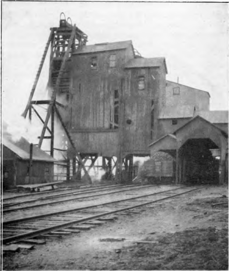
Mine tipples of Crown Hill No. 1 (in foreground) and No. 3 (in background). No 3 is one of the best equipped mines of the county.
