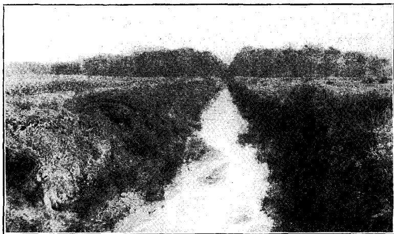
One of the large drainage ditches which are frequently seen both in Laporte and St. Joseph County.
