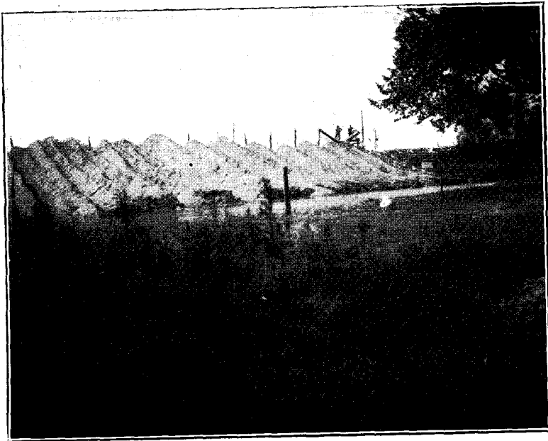
FIG. 6. Gravel dipped by means of buckets attached to an endless chain. Near Fountain-town, Shelby County. (Photo by B. W. Kelly.)
