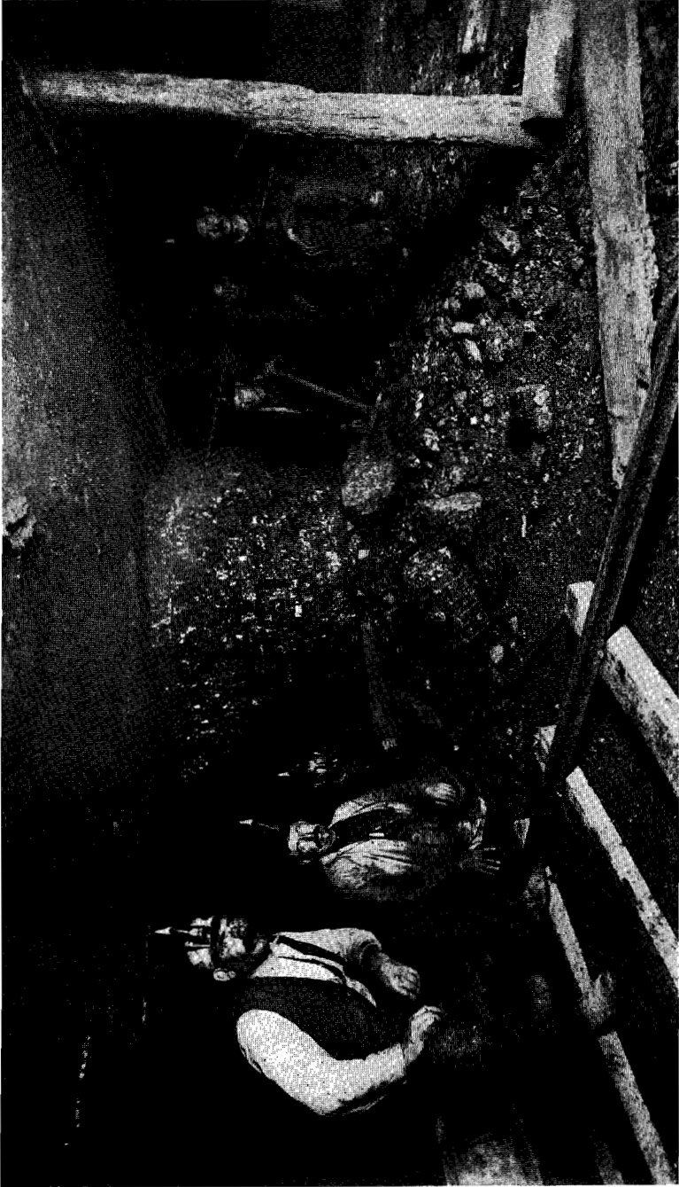
DRAWING A PILLAR IN GREEN VALLEY MINE, NEAR JASONVILLE, IND.
