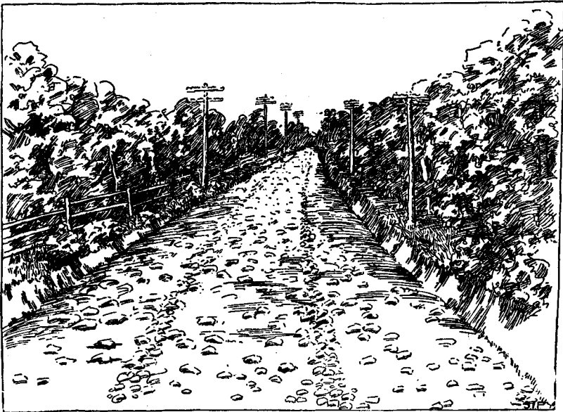
Fig. 16. Bad condition of road resulting from attempt at macadam construction with large and small broken stone. Large stones have worked out to the surface.
