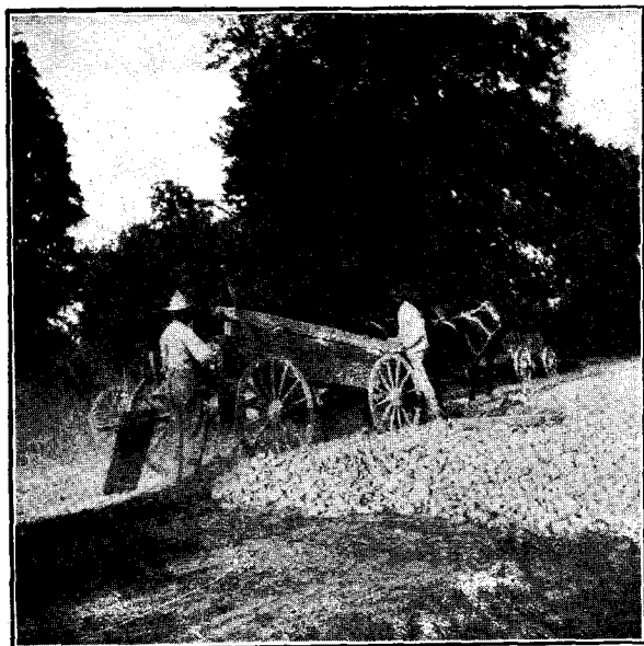
(a) Placing crushed stone on roadway east of Bloomington, Monroe County.
