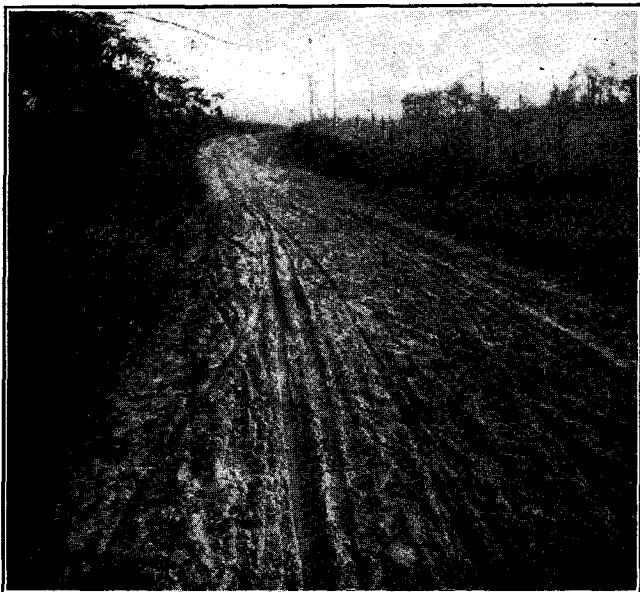
Showing that fine gravel used as top dressing for stone on steep grades is soon deposited at foot of hill.
