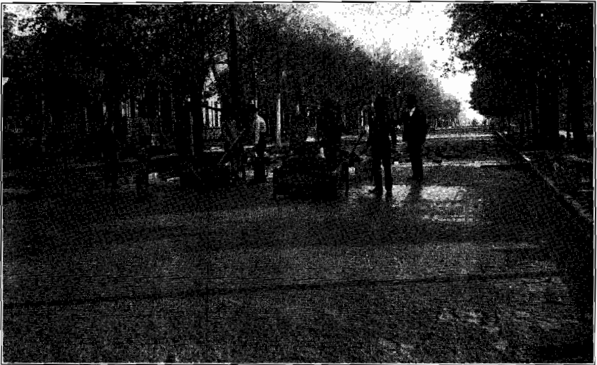
Applying the Filler.
