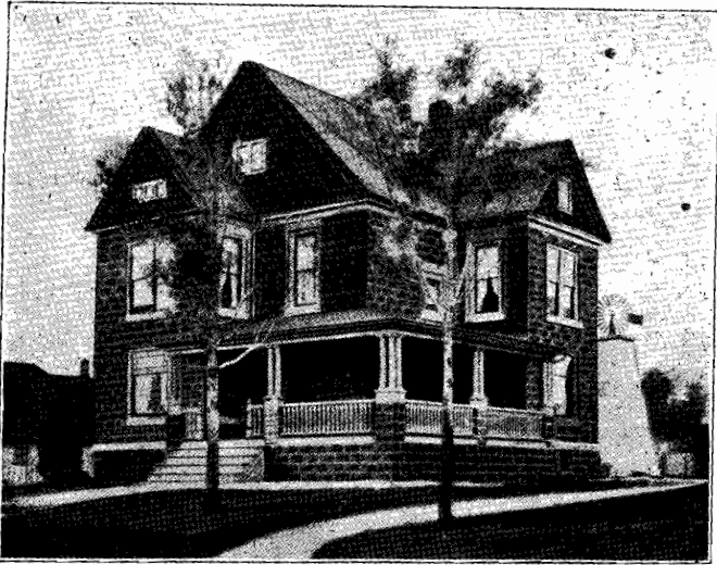
Residence constructed of Rock-faced Hollow Block.
