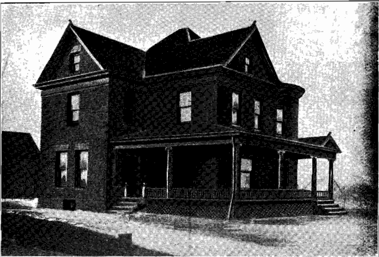
Residences made of rock-faced vitrified brick; the upper one that of I. G. Poston, Crawfordsville, Ind.
