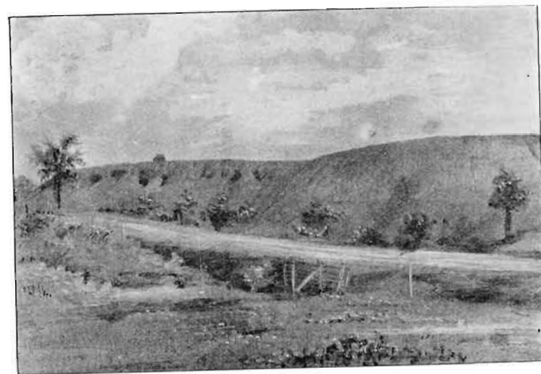
Fig. 985. Slack pile at Ehrlich mine at Secleyville, Vigo county. Extends back to tipples, of which the top just shows in distance on left side. Showing enormous volume of waste (fine coal, etc.) by former methods of mining and preparing coal for market.
