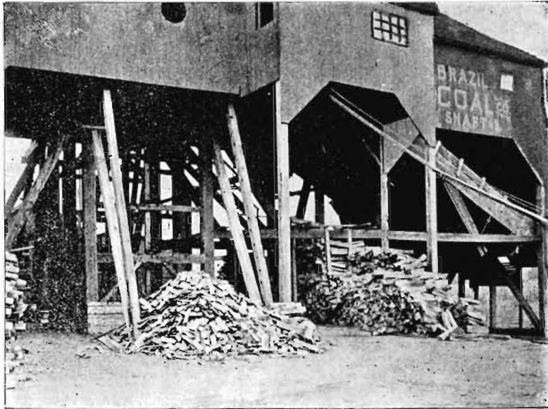
Fig. 954. Cut showing top of shaft after being equipped.
