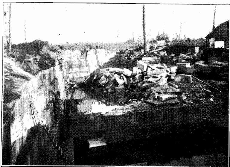
1. VIEW LOOKING SOUTH IN THE STAR QUARRY.
