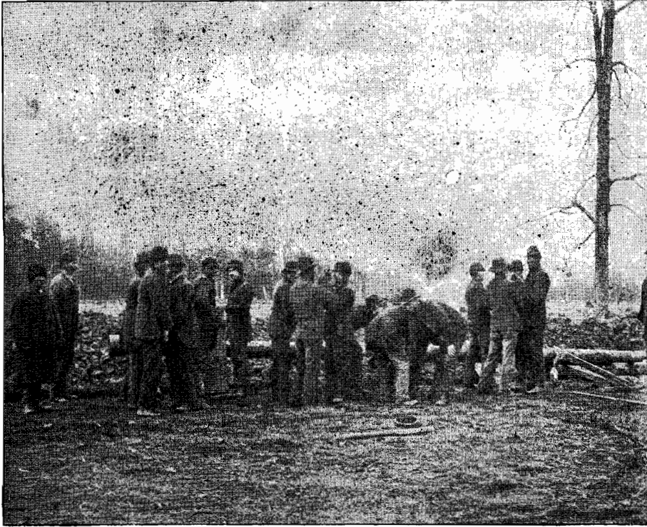
Screwing 8-inch pipe joints by hand.
